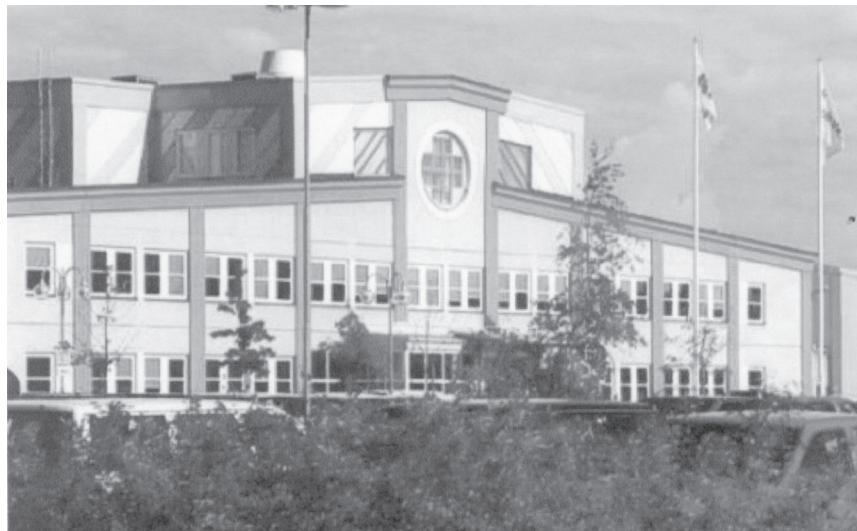
Figure 11.6. Office complex built of X-concrete elements. [20]
