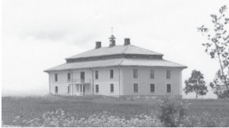
Figure 11.7. Office complex built of X-concrete elements. [20]
