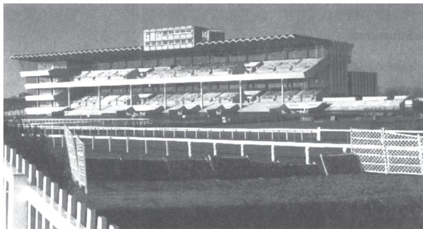
Figure 11.21. Racecourse Grandstand, Doncaster. [22]
