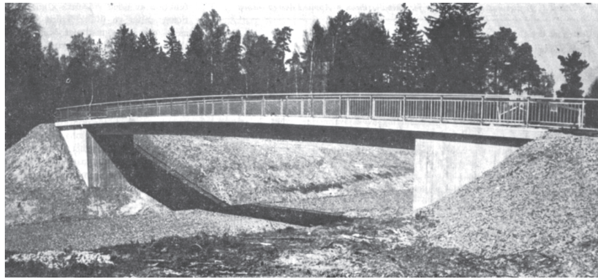
Figure 11.4. Sweden's first lightweight aggregate concrete bridge. [19]
