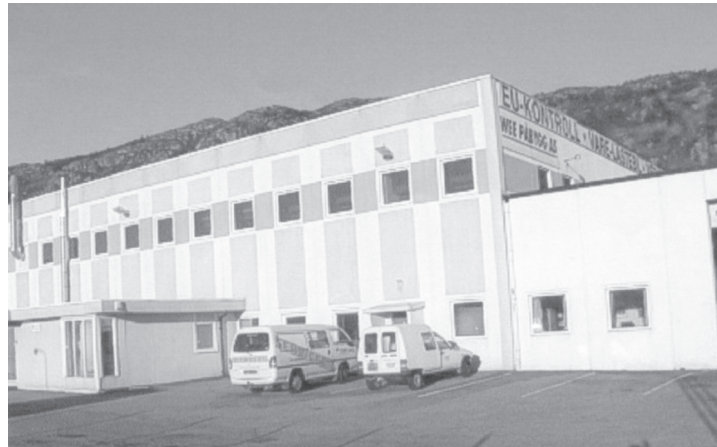
Figure 11.12. Industrial premise built of X-concrete, Norway. [20]
