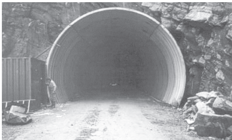
Figure 11.13. Tunnel built of X-concrete elements, Norway. [20]
